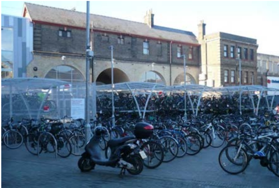
Figure 4.5: Cycle parking at Chelmsford Station
