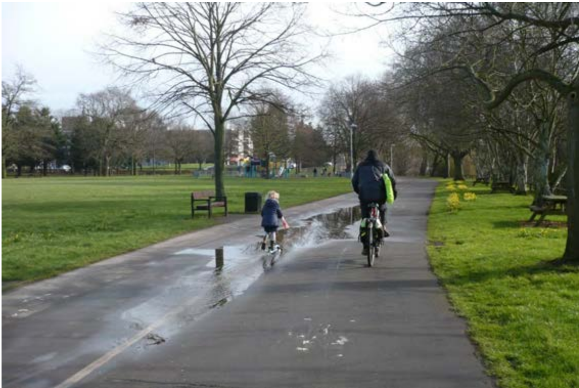
Figure 4.2: Drainage issues in Central Park
